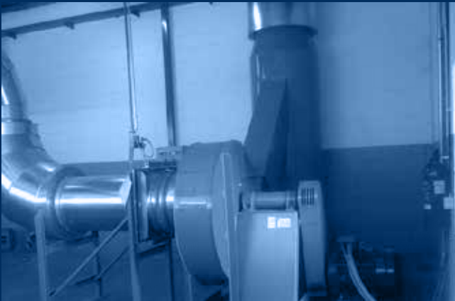
vista ventilatore Atex / Atex fan view
