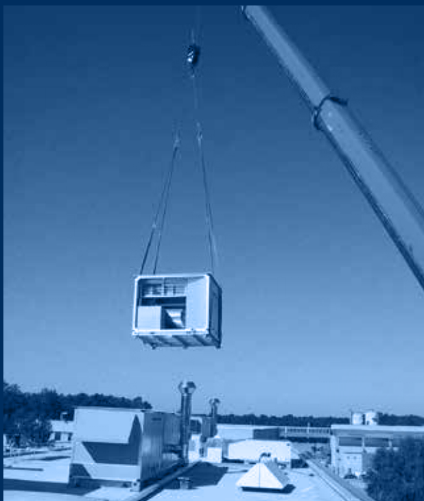
vista roof-top /roof-top view
