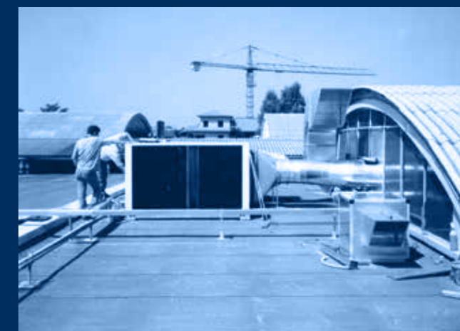
vista macchina in copertura / plant's view on the roof
