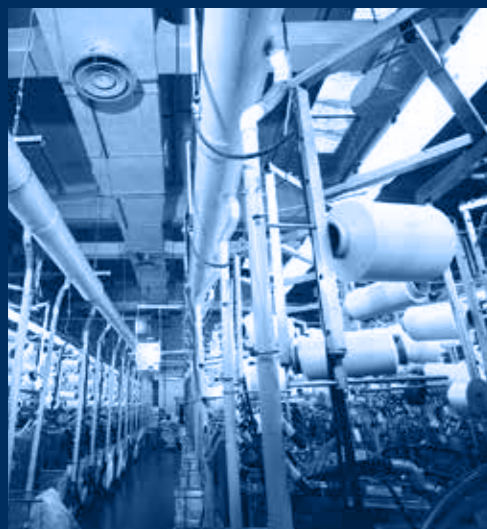
interno tessitura / inside of weaving department
