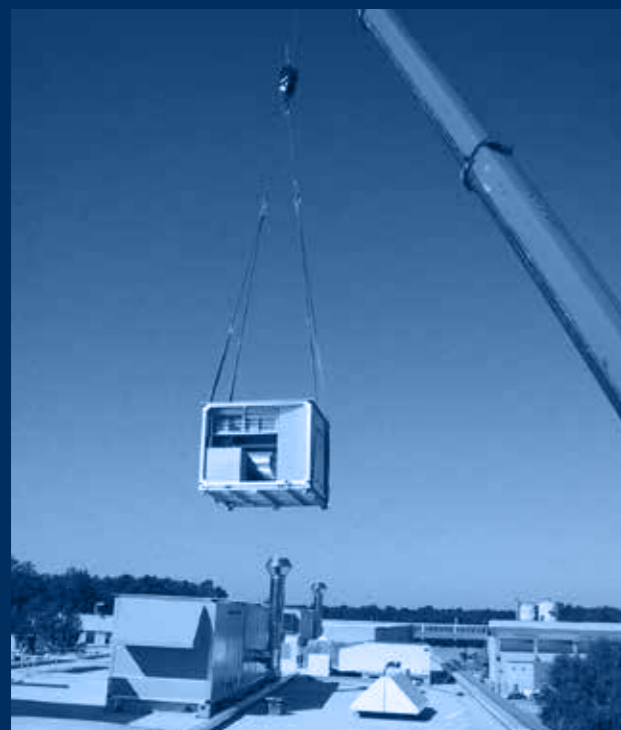
vista roof-top / roof-top view
