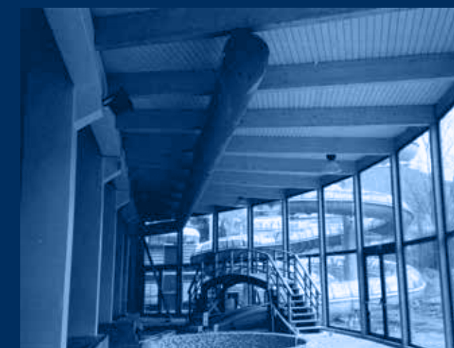
vista canale immissione in tessuto zona 1/view of the fabric immission channel in zone 1
