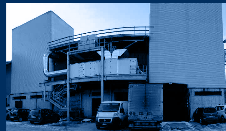
vista globale esterna impianto /external global view of the plant
