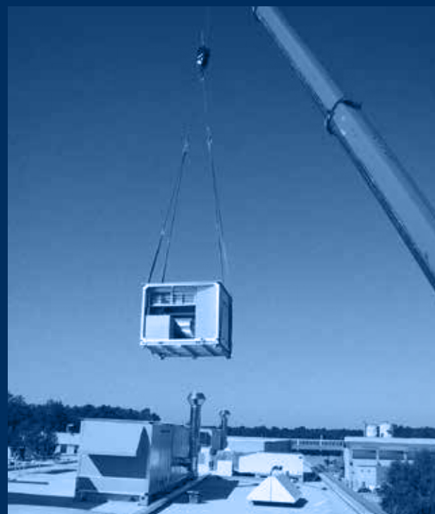
vista roof-top / roof-top view
