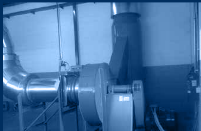
vista ventilatore ATEX / ATEX fan view
