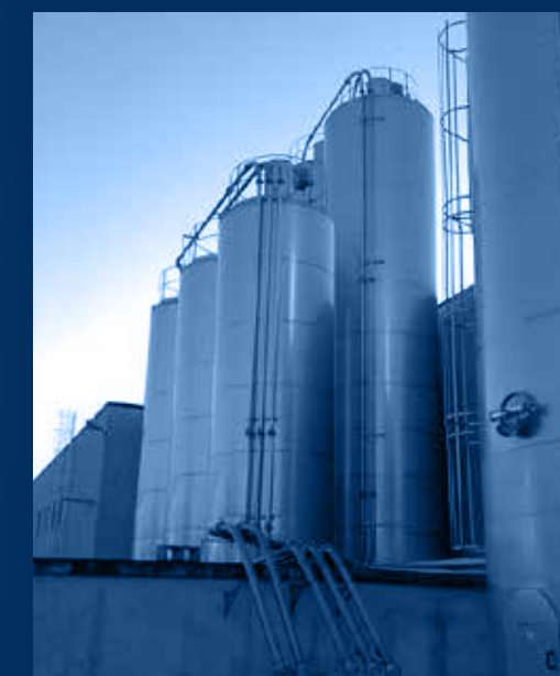
vista frontale sili / frontal silos view
