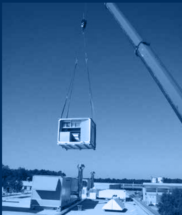
vista roof-top / roof-top view
