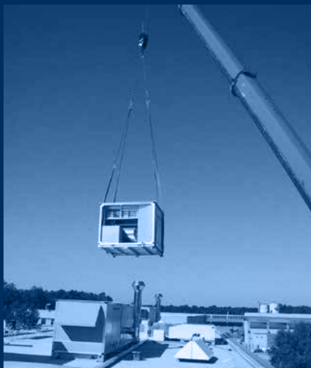
vista roof-top / roof-top view
