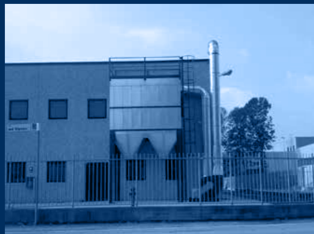
vista filtro depolveratore a maniche /sleeve filter view
