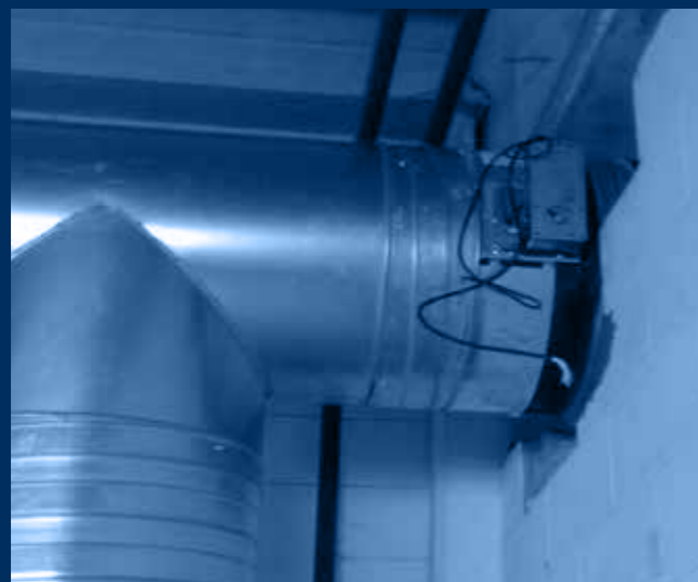
vista serranda tagliafuoco in attraversamento reparto / fire damper view in wall crossing between departments
