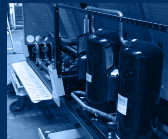
vista circuito frigorifero / refrigerant circuit view
