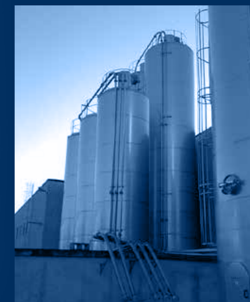
vista frontale sili / frontal silos view
