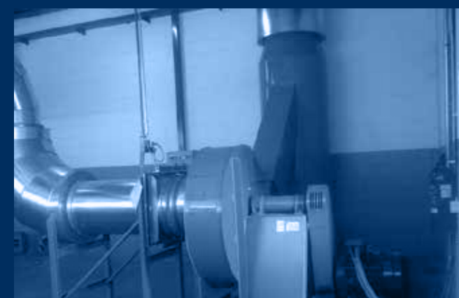
vista ventilatore ATEX / ATEX fan view
