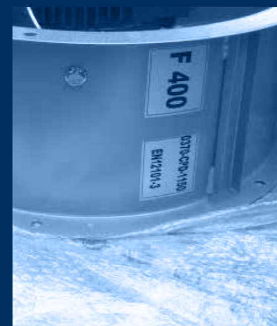
vista evacuatore forzato 400°C/2 h / extraction fan 400°C\2h view
