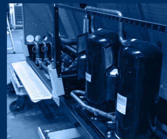
vista circuito frigorifero / refrigerant circuit view
