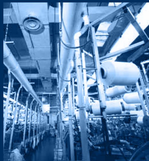
interno tessitura / inside of weaving department
