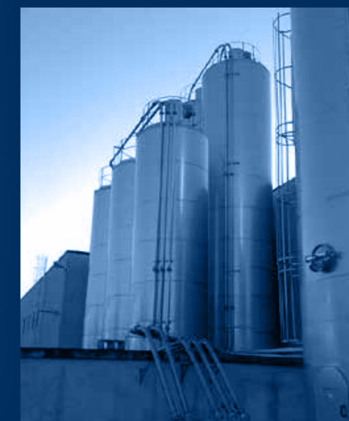
vista frontale sili / frontal silos view
