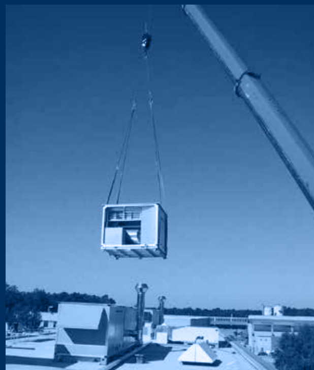
vista roof-top / roof-top view
