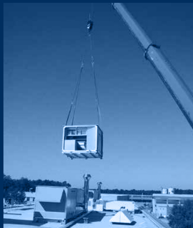
vista roof-top / roof-top view
