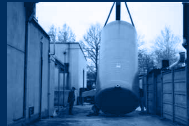
serbatoio in vetroresina 20.000 lt / plastic (reinforced with fiber glass) tank 20.000 lt
